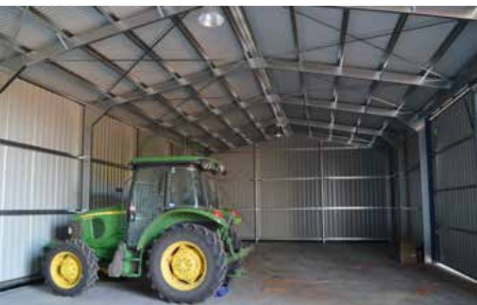
Inside Ashley's new 9m span shed. Note the bracing in the roof which adds significant strength.
