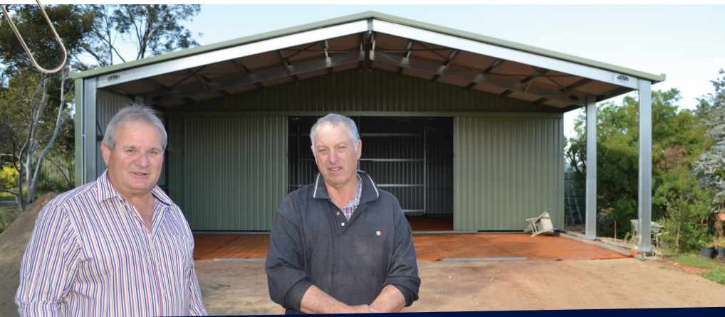
Barry Williams of Murray Bridge (right), pictured here with Grant Sheds owner Danny Halupka , is delighted with his new 12m x 15m x 3.6m shed. It is 12m span with a 9m deep enclosed area at the back to securely protect Barry's "toys" like his caravan, cars and trailer. The front Garaport section gives him a huge entertaining area in his back yard and additional undercover parking area.
