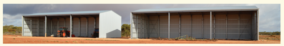
12m x 27m x 6.3m Machinery Sheds Two of the three identical sheds that the Byrne Group of farms & vineyards purchased. Each has 3 x 9m wide bays for easy access for wide machinery or for hay storage.
