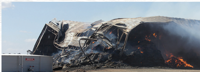
Hundreds of sheds burnt down in the Pinery bushfires. The fire fighting water storage tank on left was no help under these catastrophic circumstances. Photo courtesy ABC web site
