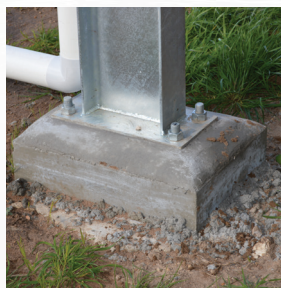
Solid UB, hot-dip galvanised columns & footings bolts for secure anchoring.
