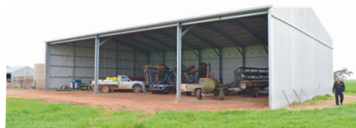
This 2004, 15m x 24m x 5.1m Machinery Shed with 2 x 9m and 1 x 6m wide bay beams was unharmed in the fire.
