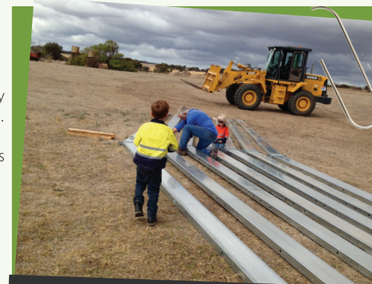
Lewis Bennett's grandsons Ned & George help him bolt shed framing together
