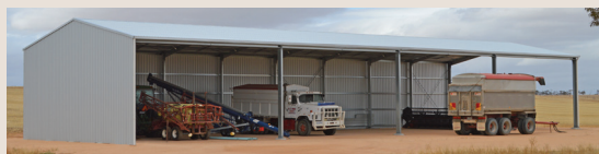
Bob's Grant Sheds Machinery Shed built in 2013. 12m x 36m x 5.1m, open 1 end & 1 side. 3 x 9m beams on the open side.
