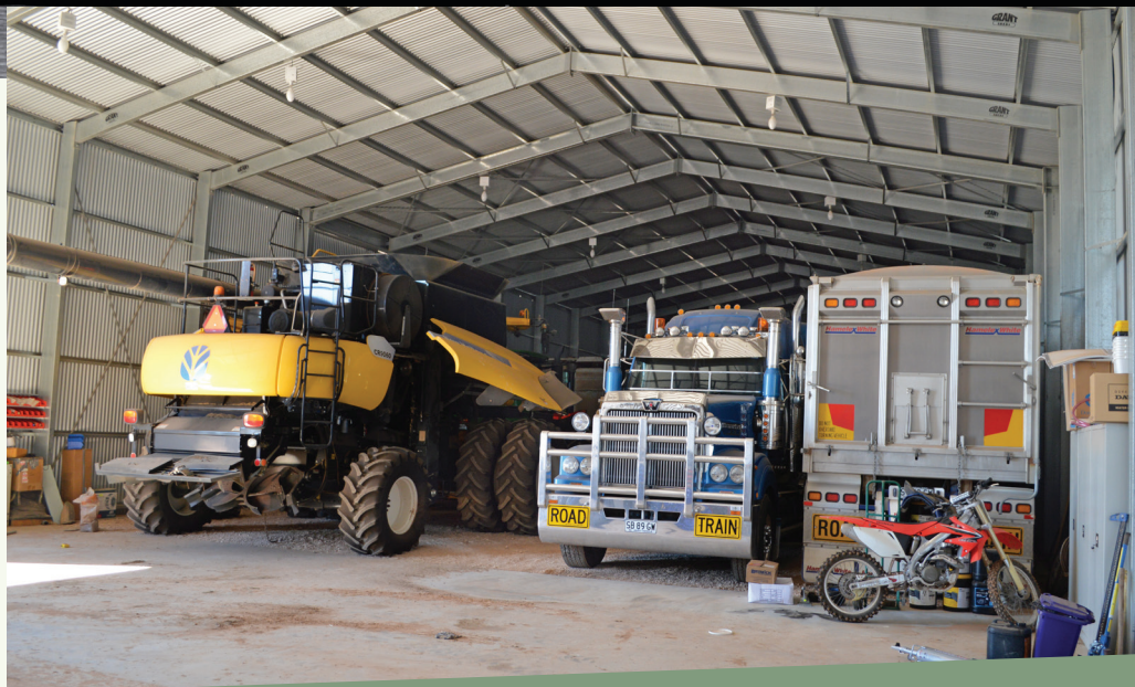
Inside Greg (Cudjee) Warmington's 15m x 45m x 6.3m Grant Sheds Machinery Shed. And at top: Todd Warmington, Danny Halupka of Grant Sheds and Greg 'Cudjee' Warmington.
