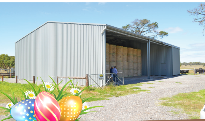
This 15m x 22.5m x 5.1m Grant Sheds hay shed has 2 x 9m beams to provide wide clear openings and has an additional 4.5m wide lock-up bay with easy-glide sliding door at the far end.
