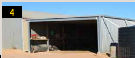
4 Leanto—9m x 24m x 3.9m Attached to existing shed
