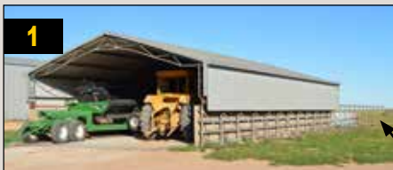
1 150 tonne Sliding Roof Bulk Fertiliser Shed Note framing behind shed where roof will roll to when opened for semi tipper access
