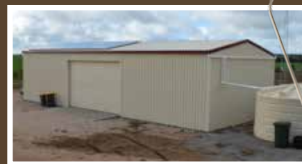
7.5m x 18m x 3.6m Home Garage
